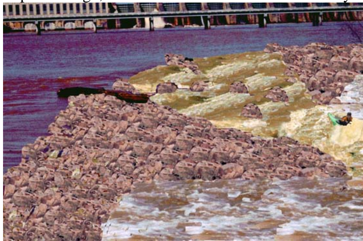
Conceptual design with wider intake area, with the weir not spilling, and natural rock added to the weir for appearance.
