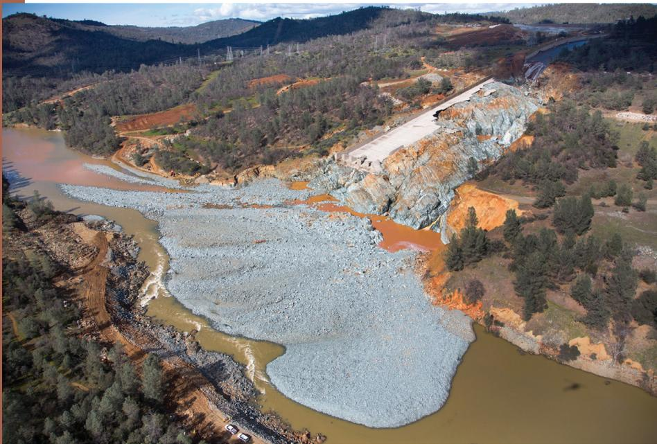
Debris in the Feather River below Damaged Main Spillway. Source: Dale Kolke, DWR.
