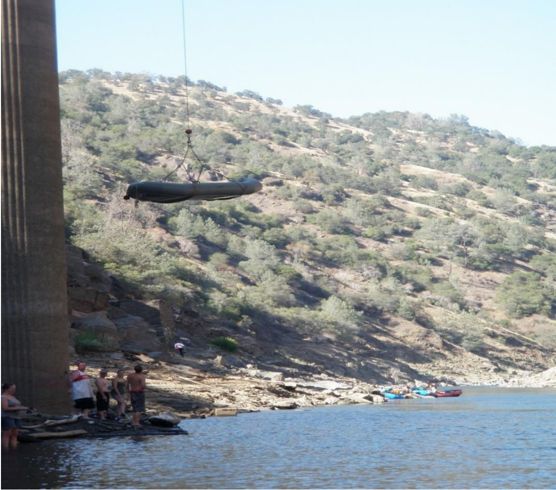
Figure 7. Booming rafts on the bridge is a safety concern for the public.
