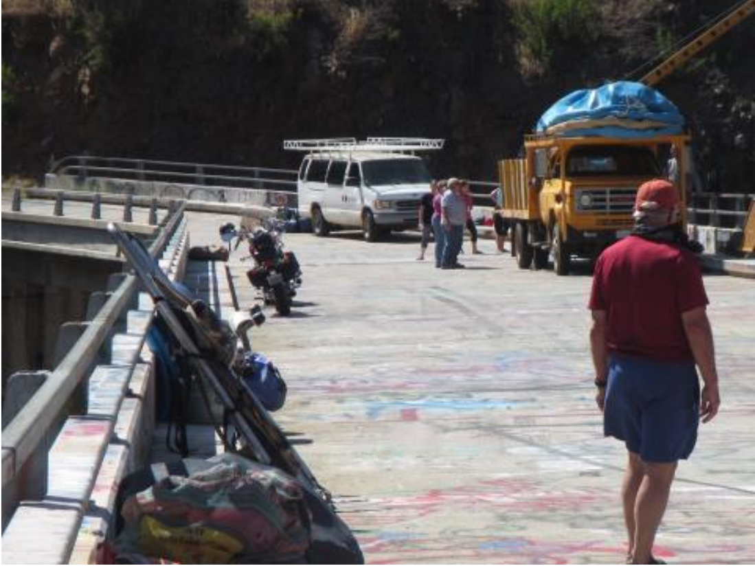
Figure 5. Demonstrates pedestrian safety concerns on the bridge.
