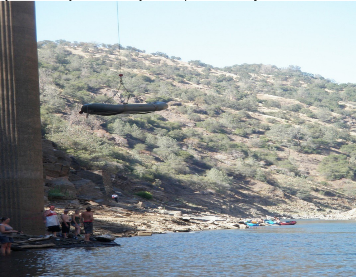
Figure 5. Booming rafts on the bridge is a safety concern for the public.
