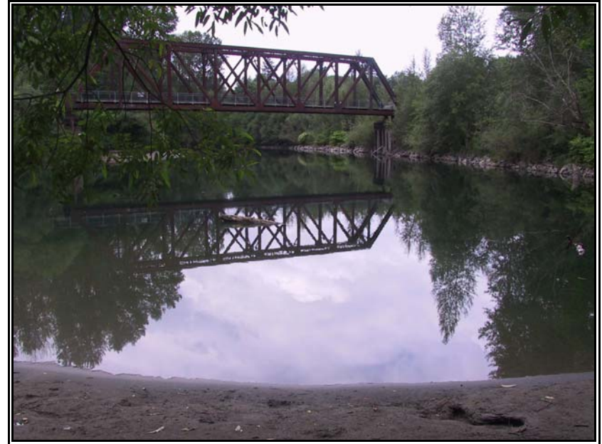
Meadowbrook Bridge site
