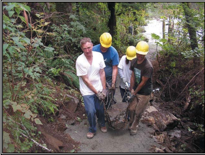
Volunteers haul rock to improve a trail at the Mine Creek site.
