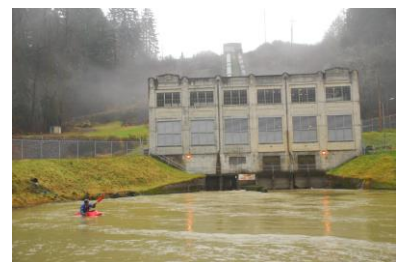
Nisqually Park at Yelm Powerhouse. Photo: Thomas O'Keefe
