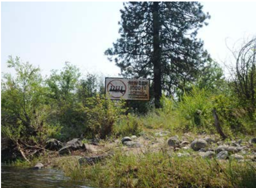
Dryden Dam, Wenatchee River, WA
