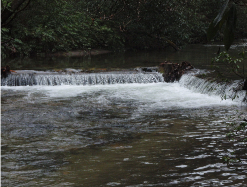
1. Human placed log v-weir on Holcomb Creek.
