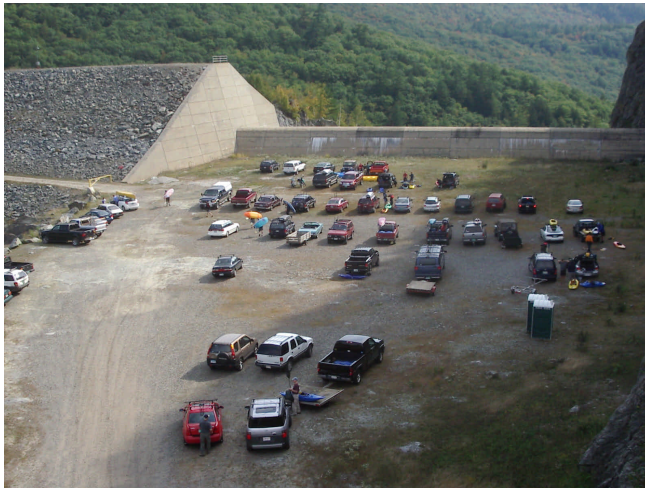
Figure 1: Ball Mountain Dam Parking Lot and Impoundment
