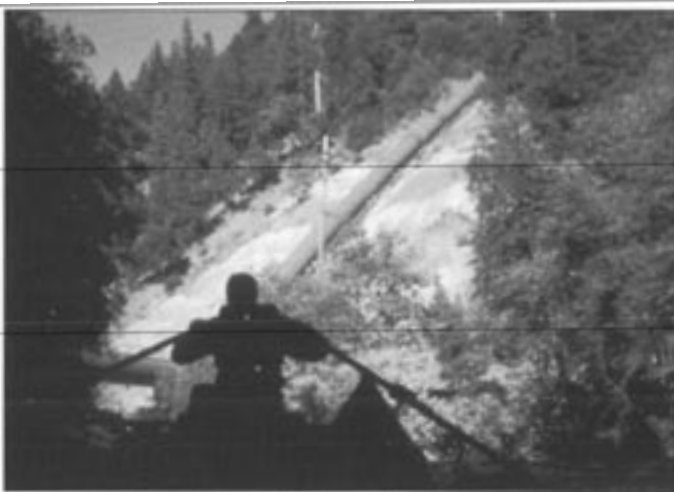
Catboater passing under the penstocks used to deliver water to the Belden Powerhouse on the North Fork Feather River. Photo John Gangemi.
