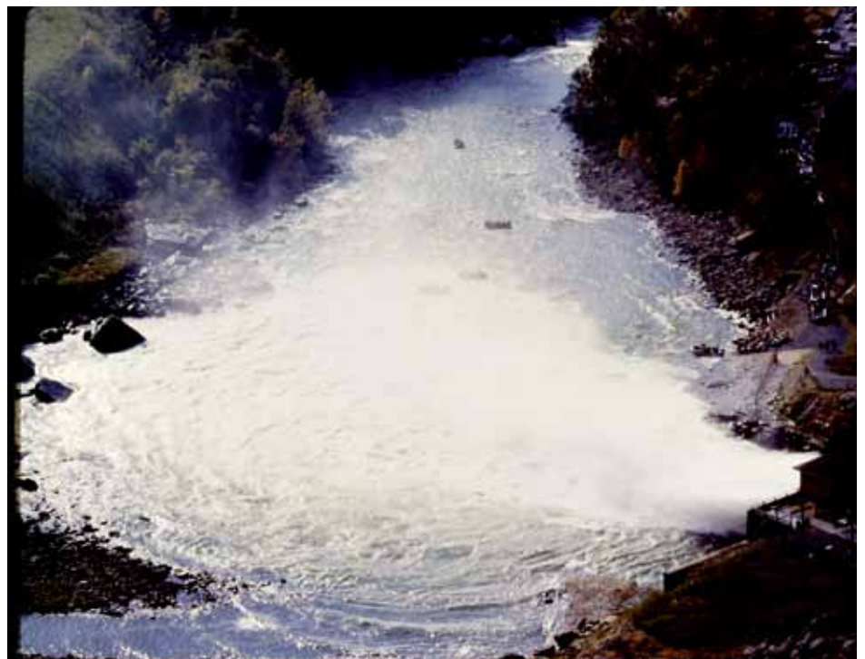
The discharge tubes at Summersville Dam Photo by Jerry Spence
