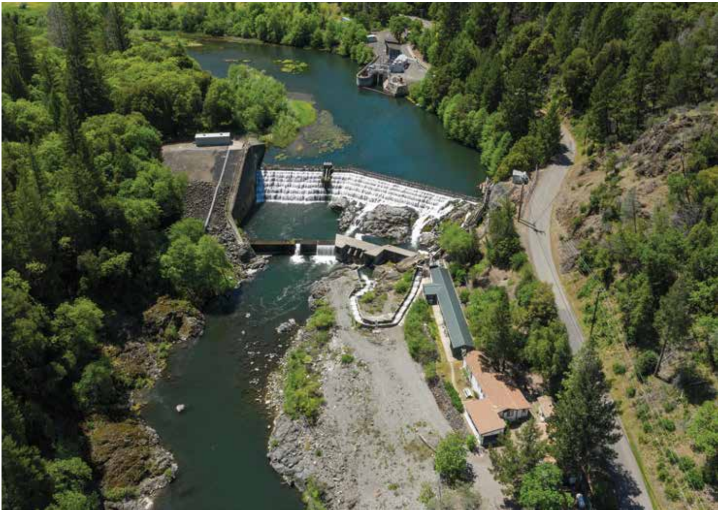
Cape Horn Dam, 62 feet tall, backs up the Eel River so it can be diverted into a tunnel. Photo: Kyle Schwartz/CalTrout
