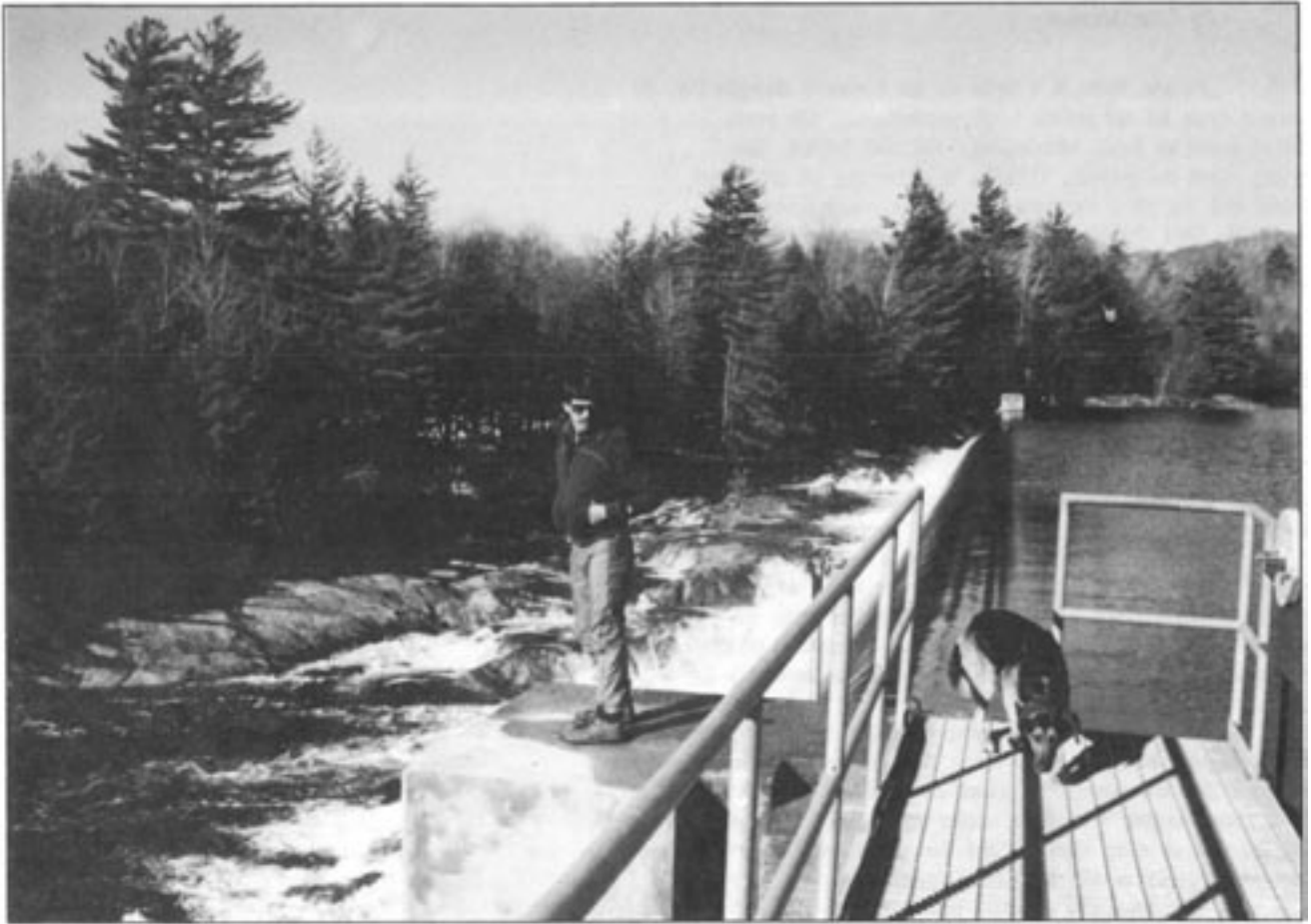
Steve Massaro and his constant companion D.O.G survey a stretch of potential whitewater below a New York hydro site. This stretch, now not utilized by New York boaters, could be reestablished with favorable relicensing.
