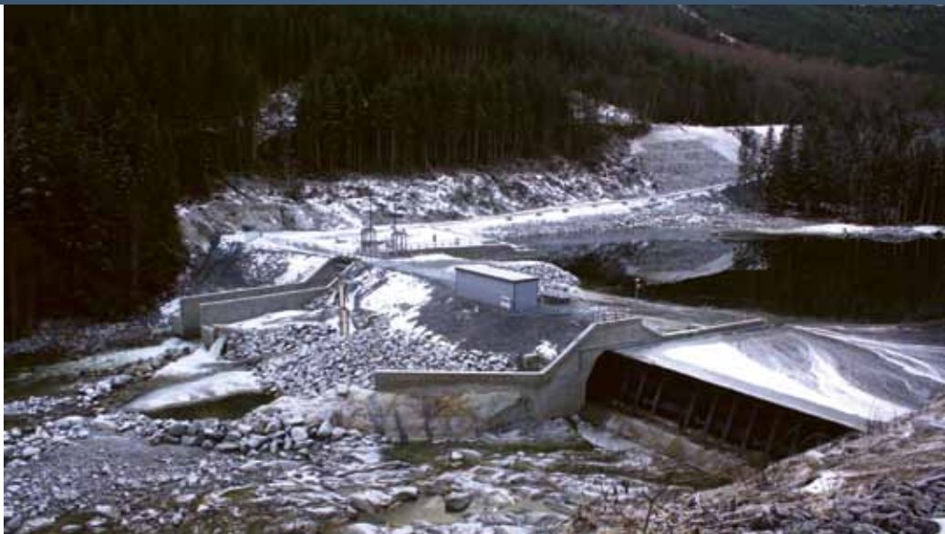
The 49-MW Ashlu Creek Hydropower Project in B.C. is an example of the type of project that California was considering for inclusion under renewable energy standards. In January 2014, the state declared that B.C. hydro did not qualify as renewable.
