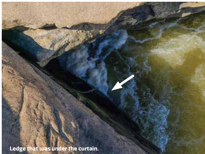
Kanawha Falls undercut hazard and safety chain. Photos: Brent Samples.
