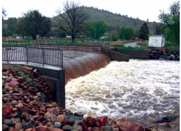
The Highland Diversion in Lyons, Colorado.
