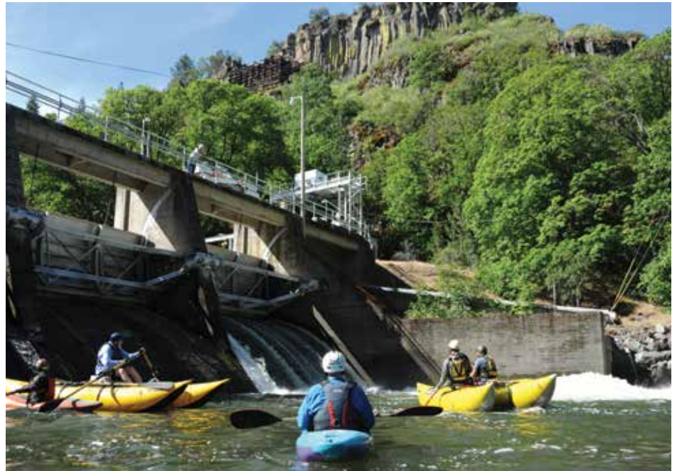
Waiting for PacifiCorp to turn on the water at the base of Copco 2 Dam prior to a test flow of Ward's Canyon Photo by Thomas O'Keefe
