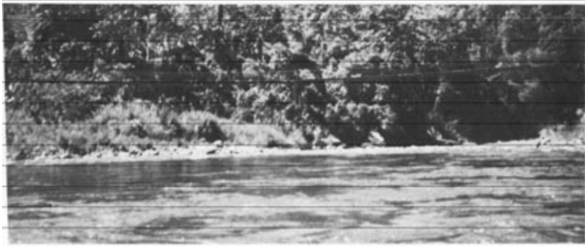
Footbridge along the Jatate River in Southern Mexico.
