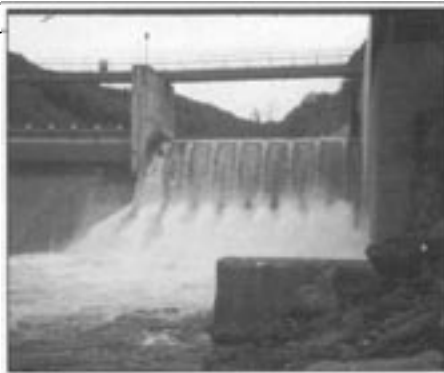
#5 Dam at Monroe Bridge, Deerfield River.
