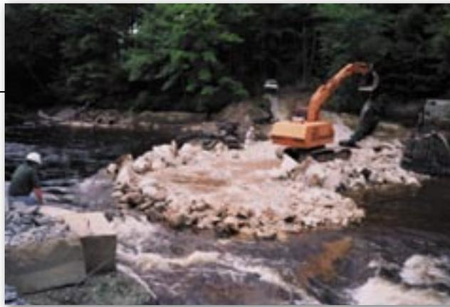
Over the next five weeks controlled blasting and removal of debris would take place, freeing up the river and exposing river features that would delight paddlers when the fall rains arrive.
